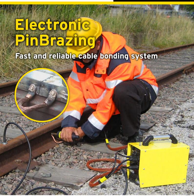
Electrical cable connection system for signaling, return current and earthing applications for the rail industry
