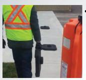
• Place rubber post bases on firm level surface at approximately 12 ft. apart (starting from cartridge) or 4 paces.
