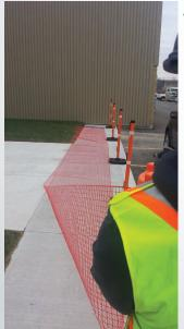
Lay fence on ground. If area is full of debris, mud or otherwise, a 2nd person can hold fence upright while retracting.
