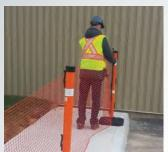
• To retract system, first remove fence from post hooks starting from end post.
